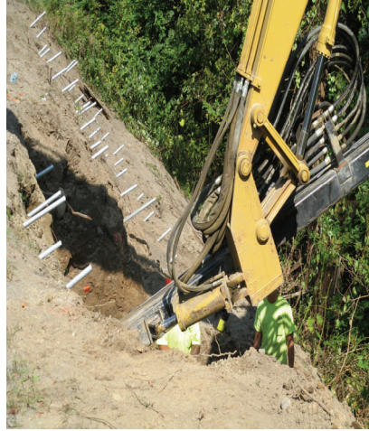
Soil Nail Launcher repairs landslide on Lincklaen Rd. in late September.
